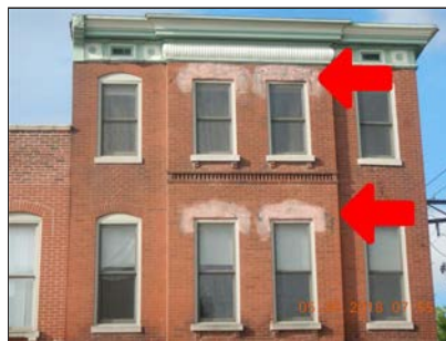
prior lintel/tuckpointing work
