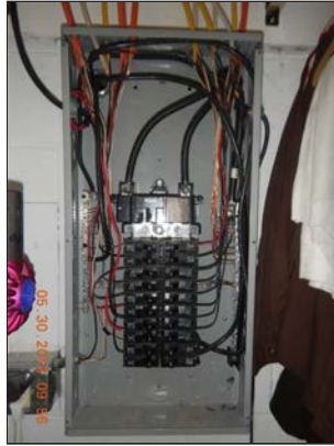
interior of this panel is in good condition
